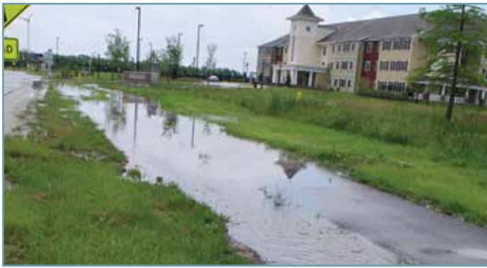
This photograph illustrates flooding to the north of Prairie Place on June 15, 2015. The CMAP Local Technical Assistance grant will provide the first comprehensive stormwater management plan for the campus since construction in 1969. This roadmap can be used in future planning as the university moves toward realization of Vision2020.
