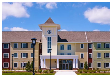
Prairie Place Residence Hall
