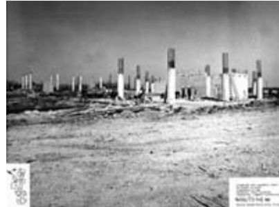
Construction of GSU, 1972
