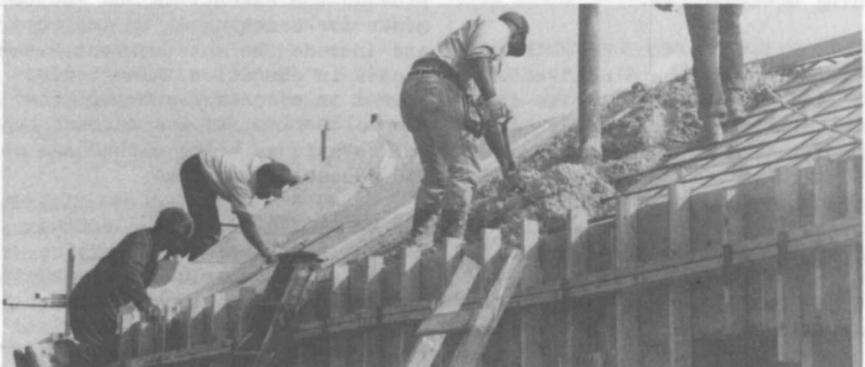
*Workmen pour and shape concrete to form the roof of "Divided House" by Bruce Nauman. Concrete valued in excess of \$5000 was contributed by the Arquilla family of Accurate Ready Mix Concrete Co., Hazel Crest.*
