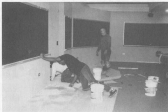
Craftsmen lay carpeting in B-wing classroom.
