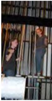
installation of new rigging ropes. Gone are the old manila ropes installed in 1995 that could only hold 4,000 lbs. and gave stagehands splinters.
